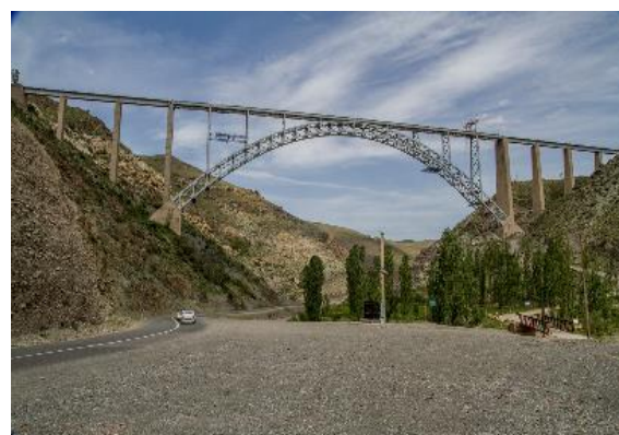
Figure 2. The long-span steel-truss arch railway bridge
