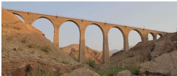
Figure 1: A view of the Shahbazan bridge.
