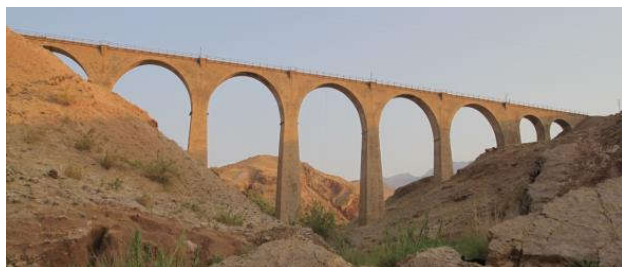
Figure 1: A view of the Shahbazan bridge.
