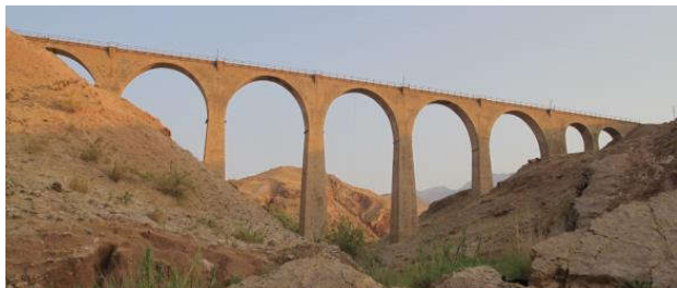
Figure 1: A view of the Shahbazan bridge.
