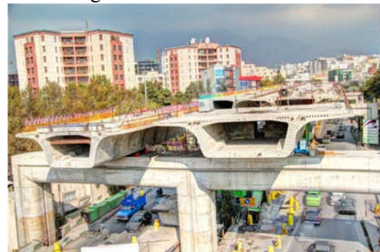
Figure 2: The Sadr Elevated Expressway, Under Construction (2012), Tehran, IRAN
