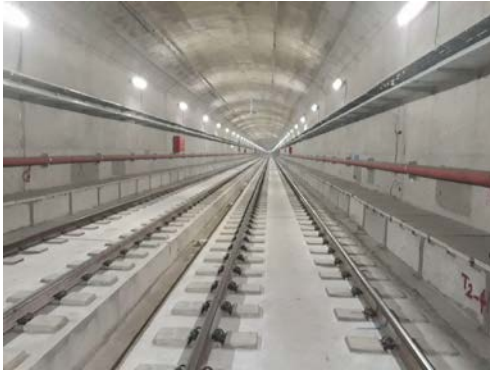
Figure 1. Test location in Isfahan city.
