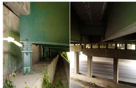
Figure 11. Use of steel deflector beams to increase clearance and mitigate collision risk
