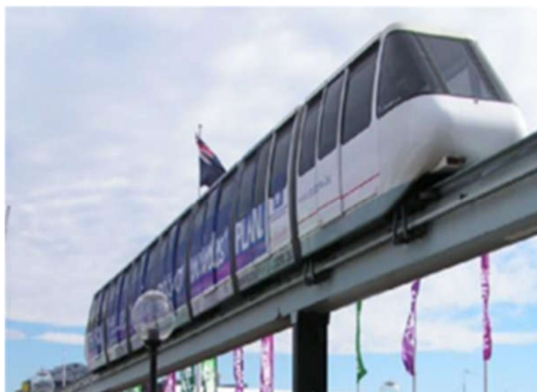
Figure 3. Monorail on its track
