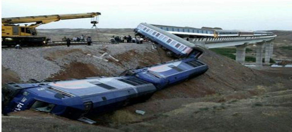
Figure 1. Derailment of the train due to rail removing (Iran 2020)
