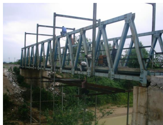
Figure 5. Overview of the Neka truss railway bridge.
