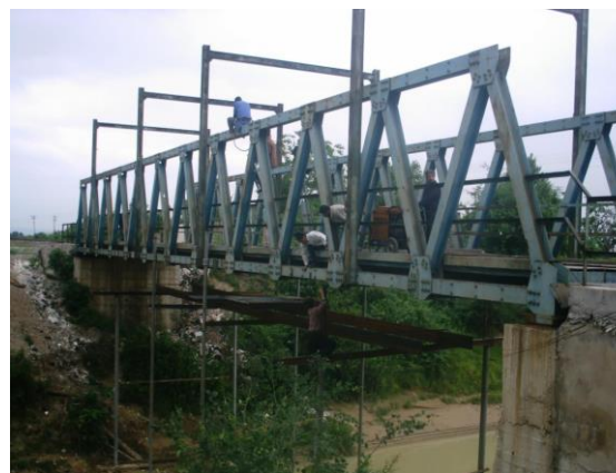
Figure 5. Overview of the Neka truss railway bridge.
