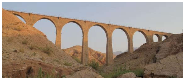
Figure 1: A view of the Shahbazan bridge
