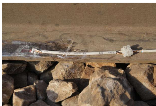
Figure 5: Strain gauge mounted on rail head to determine the exact speed and location of test train axles
