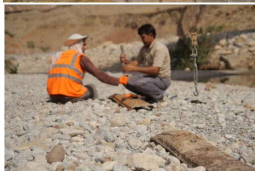
Figure 3: a) DCDT sensor mounted in the middle of the span, b) DCDT's cable fixed to the steel sleeper placed beneath the span (conventional method)
