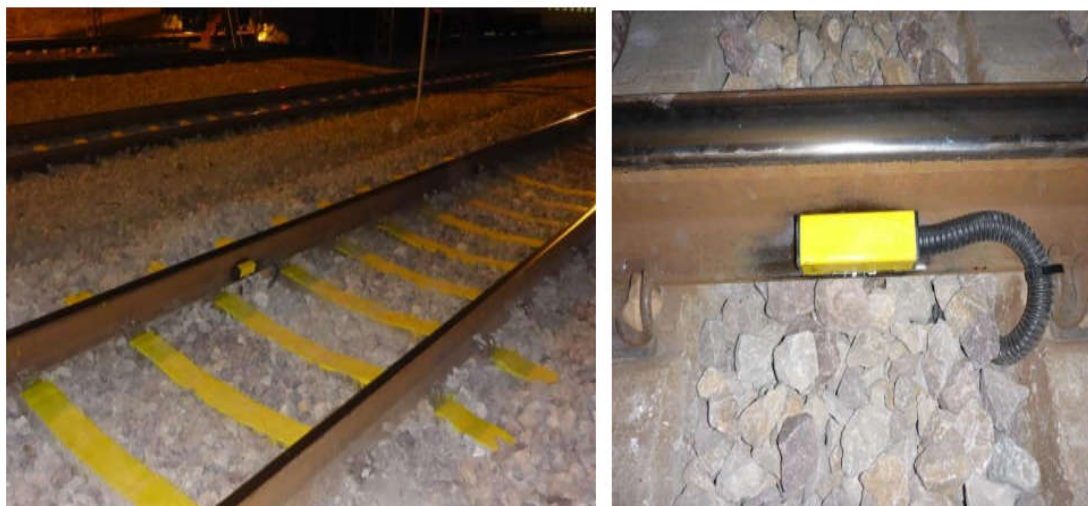
Figure 5. Protection of the sensors on the rail
