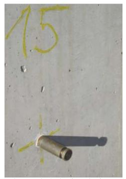
Figure 6. "Fixed point" for track reference
