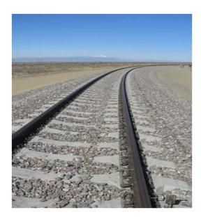
Figure 4. "Half-frame-sleeper track" (TTCI, 2009)
