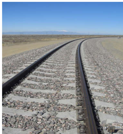
Figure 4. “Half-frame-sleeper track” (TTCI, 2009)
