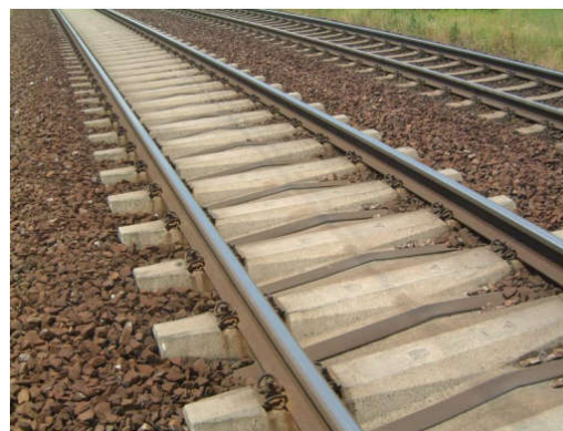
Figure 2. “Wide sleepers” (Germany, 1999)
