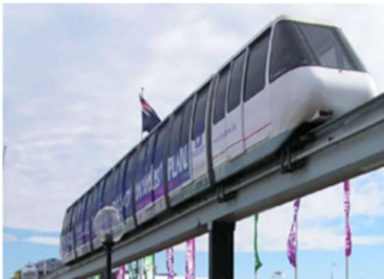
Figure 3. Monorail on its track
