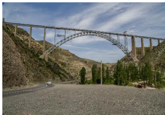
Figure 2. The long-span steel-truss arch railway bridge
