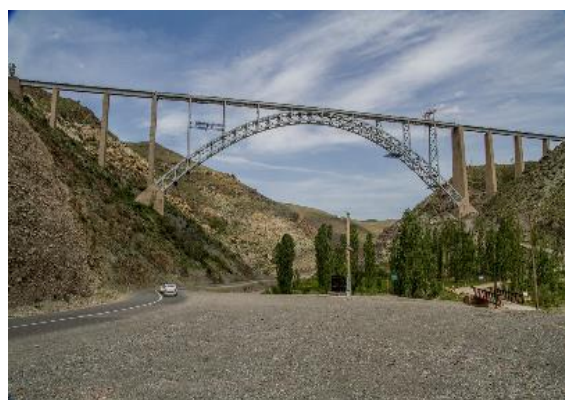
Figure 2. The long-span steel-truss arch railway bridge
