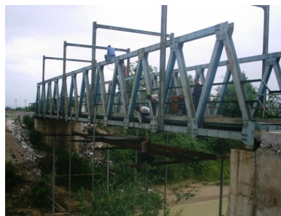
Figure 5. Overview of the Neka truss railway bridge.
