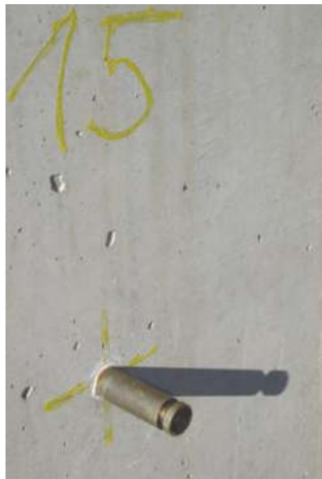
Figure 6. “Fixed point” for track reference
