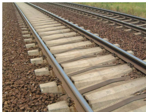
Figure 2. “Wide sleepers” (Germany, 1999)
