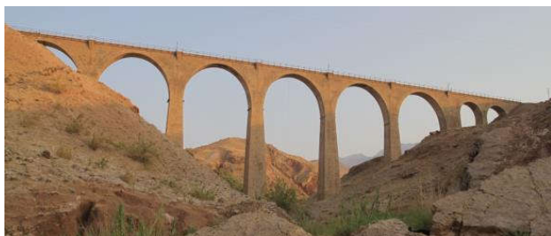
Figure 1: A view of the Shahbazan bridge
