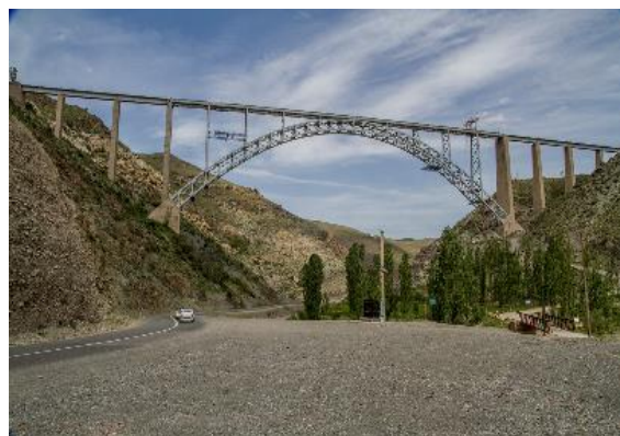
Figure 2. The long-span steel-truss arch railway bridge
