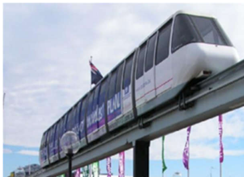
Figure 3. Monorail on its track
